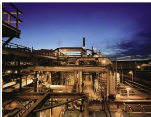
NCPPI coal to polypropylene project, Shenhua Ningxia Coal Industry, 5 x 500MW Siemens SFG-500 coal-gasifier, commissioning 2011
