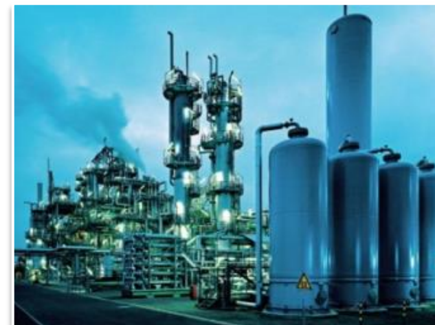
SNG-plant, CPI Xinjiang Energy Co. Ltd, Yili City Xingjiang, China, 8 x 500 MW Siemens SFG-500 coal-gasifier, commissioning 2014
